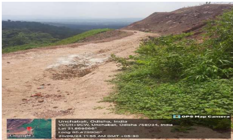
Retaining wall and Garland drain provided at the toe end of the dump
